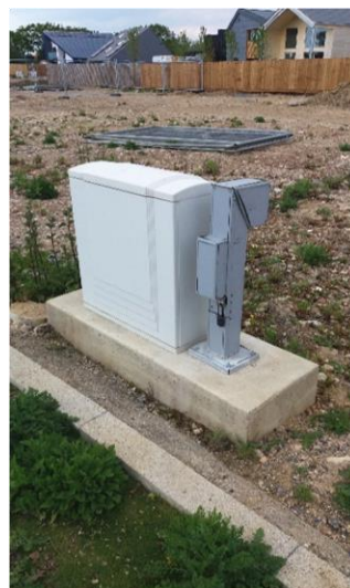
An example of services/utilities provision at Graven Hill, Bicester providing ease of access for self-builders/contractors. Service boxes are then removed post-construction
